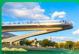
Floating Bridge Moscow
